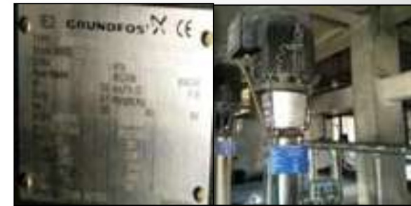
Boiler Feed water Pump
