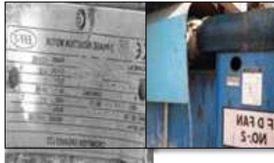
Solid Fuel Boiler FD Fan
